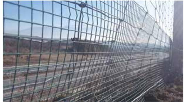
**Fig. 4.** Close-up of the fences constructed at Lot 1 of the Struma Motorway. The fine net is buried deep in the substrate and firmly fixed at the basis of the standard rabbit fence
