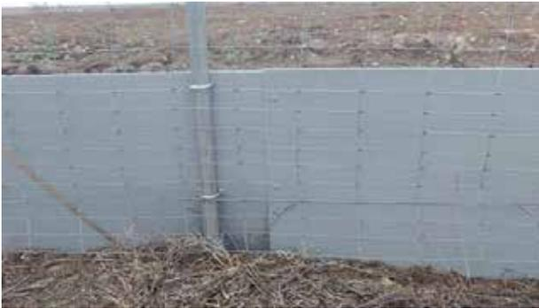
**Fig. 3.** Glass Fiber Reinforced Polymer (GFRP) plates used as barrier for preventing vehicular turtle mortality at the "Trakiya" motorway. Note the stable mounting of the plates to each other and to the metal pole
